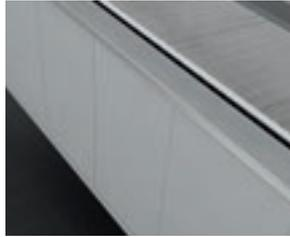
Grey powder coated sheet steel cladding (RAL7036)
